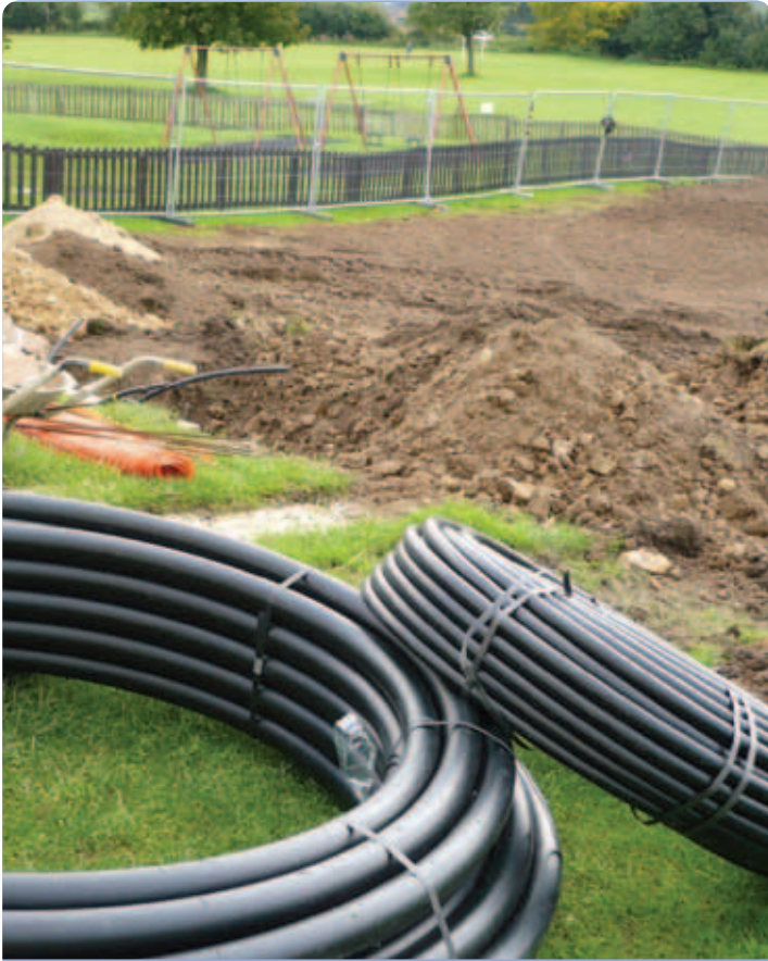
Ground source heat pump installation
