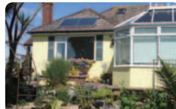
Solar water heating, Bridport (Jim Shearman)
