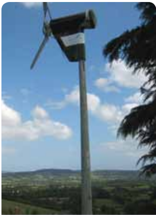
A 2.5kW Proven wind turbine Marshwood School, Dorset
