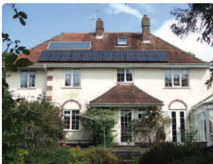
House in Bridport with solar PV and solar water heating (Photo: Jim Shearman)
