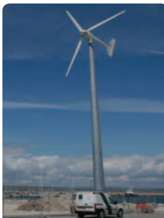
20 kW wind turbine, Dorset
